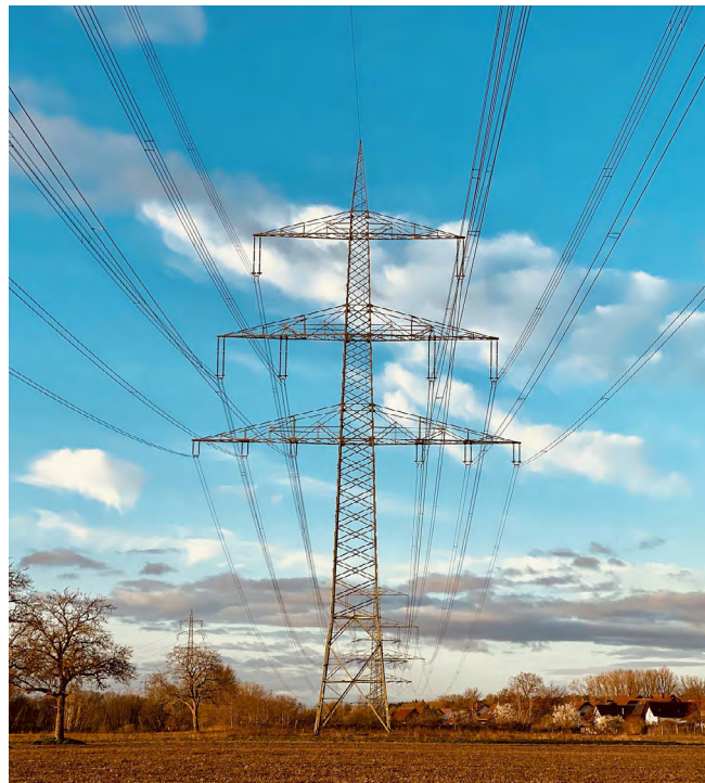
High-voltage transmission towers have relatively small footprints, though the land area beneath transmission lines is considerably greater. In assessing transmission land use, some scholars count only the footprints of the towers, while others calculate the area of the rights-of-way along the route.
