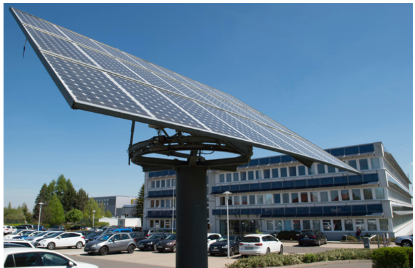
The former Solarworld facility in Freiburg, Germany. Solarworld filed for insolvency in 2017.
