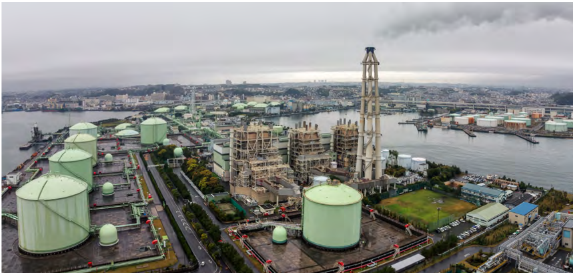
U.S. natural gas exports to Japan quadrupled between 2017 and 2019; natural gas now provides over one-third of Japan’s electricity. This is a natural gas-fired power plant in Yokohama.
